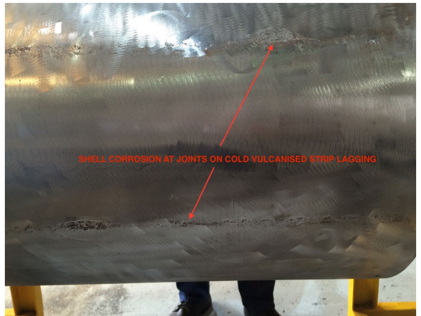
Photo #20. Pulley shell pitting from corrosion due to water ingress between lagging strips.
