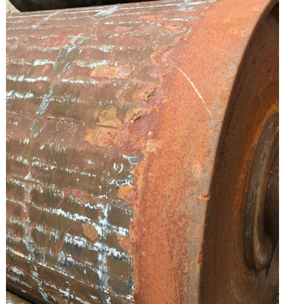
Photo #11. Failed pulley with cold vulcanised lagging removed to show edge corrosion residual adhesive pattern.
