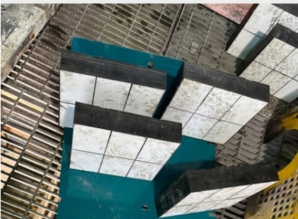
Top floor install
