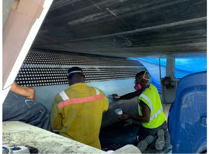
Elastotec ceramic lagging being applied on conveyor with Elastotec supervision and training
