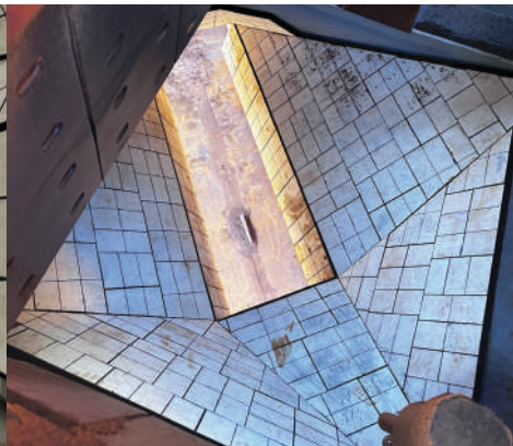
Installed Magnefast™ ceramic liners
