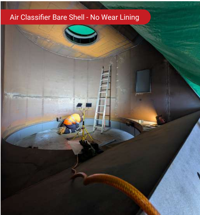
Air Classifier with Corrosion Resistant Primer
